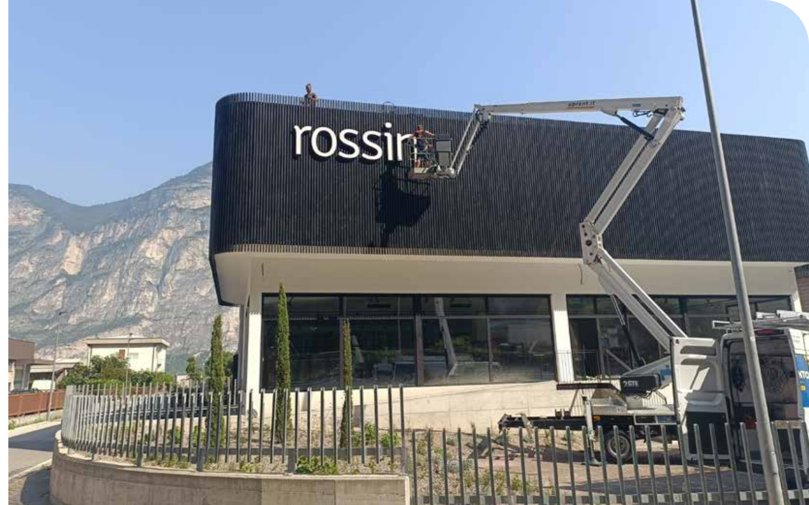
A special moment: installing the company logo on the new building.
